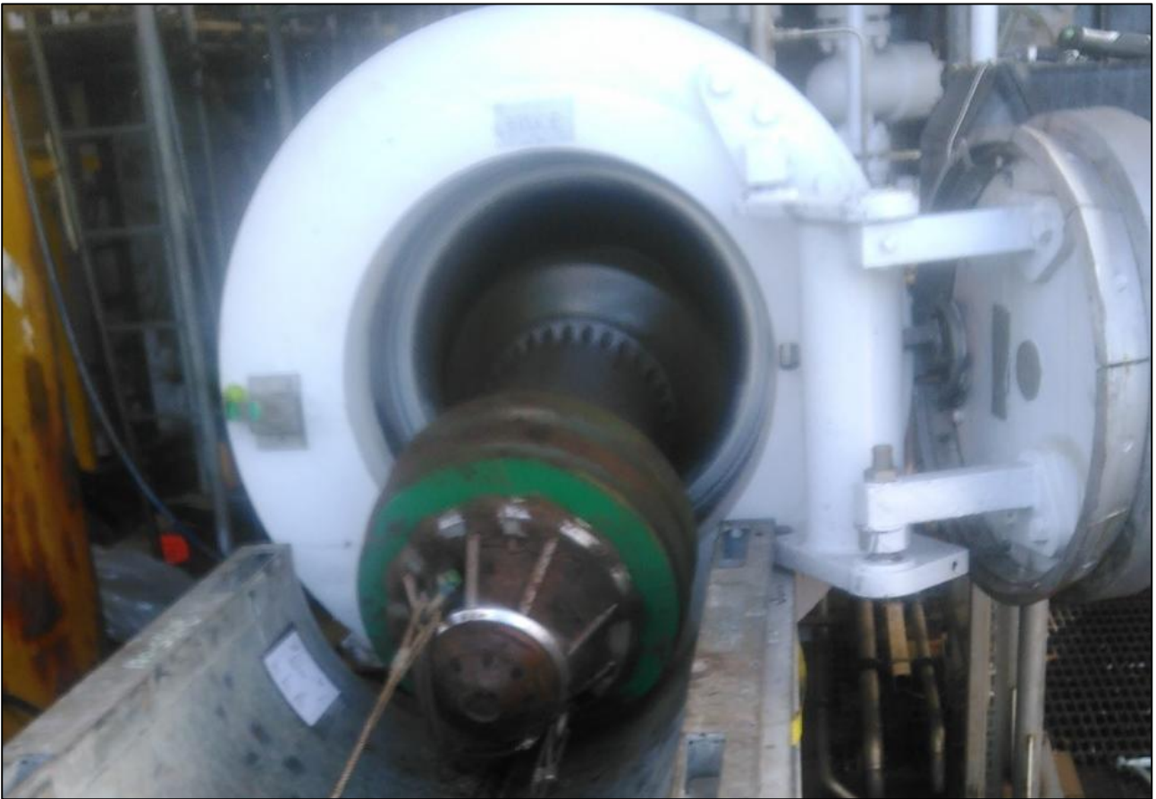
Figure 5-4 ILI tool recovery
